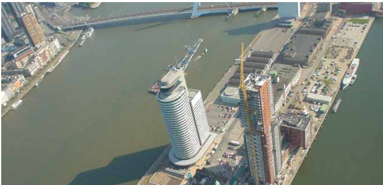
ABOVE: The Port of Rotterdam
